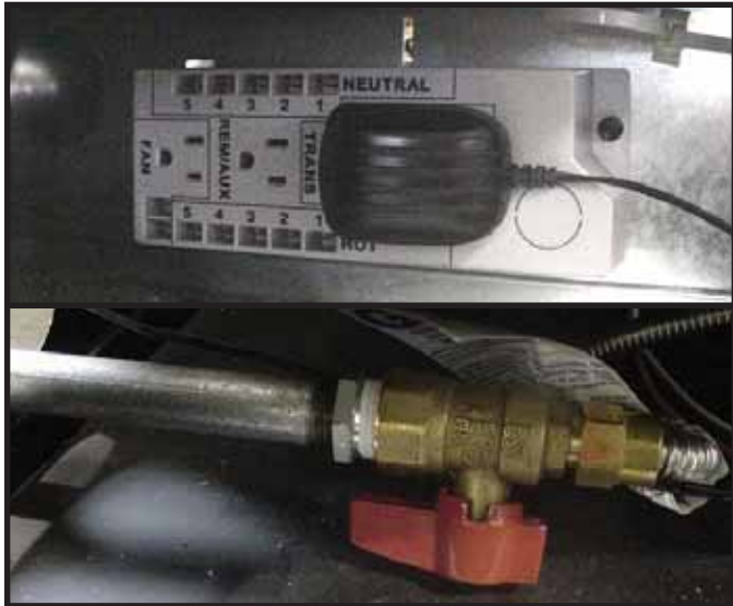
Figure 13.1 Preparation to Install Splatter Guard
